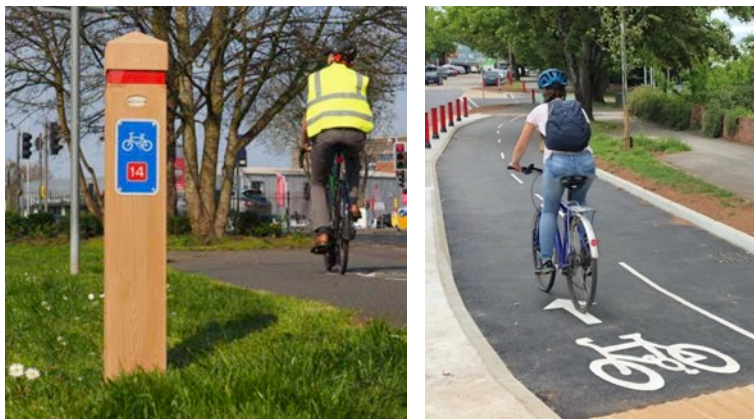
Figure 45: Left, timber-effect post that requires minimal maintenance (Glenwood 170 post). Right, painted signage on the path (Devon). Source: Glasdone www.uk.glasdon.com and Devon County Council).
