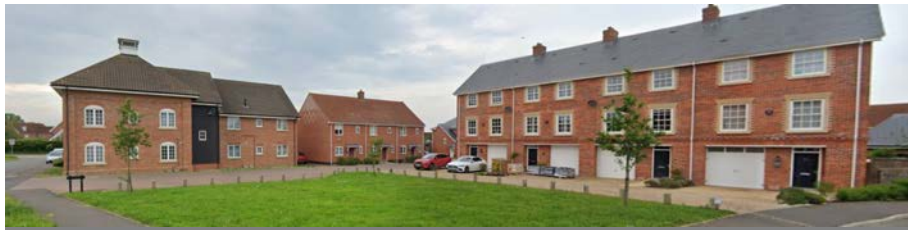
Figure 35: Varied roof heights and pitches. Mulbarton, Norfolk. Source: Google Maps, Street View.
