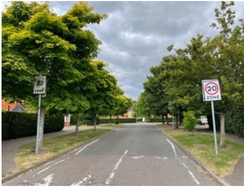
Figure 43: Tree lined road in established Rackheath. Eva Road, Rackheath, Norfolk. Source: own.
