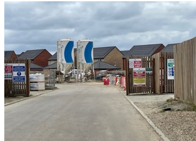
Figure 102: Construction site in Rackheath. Salhouse Road, Rackheath. Source: Own.
