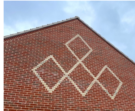
Figure 30: Diapering, brick detailing adds interest to an otherwise blank wall. Mulbarton, Norfolk. Source: own.
