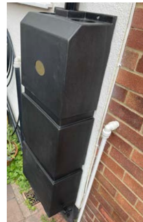
Figure 70: Discrete residential water butt for small property. Norwich. Source: own.
