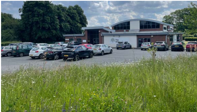
Figure 89: Community car park to serve the Willow Centre (community centre) and adjacent primary school, enabling capacity at peak drop-off and pick-up times. Cringleford, Norwich. Source: own.
