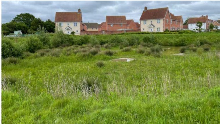
Figure 67: Wetland SuDS, providing a green entrance to the development. Mulbarton, Norfolk. Source: own.
