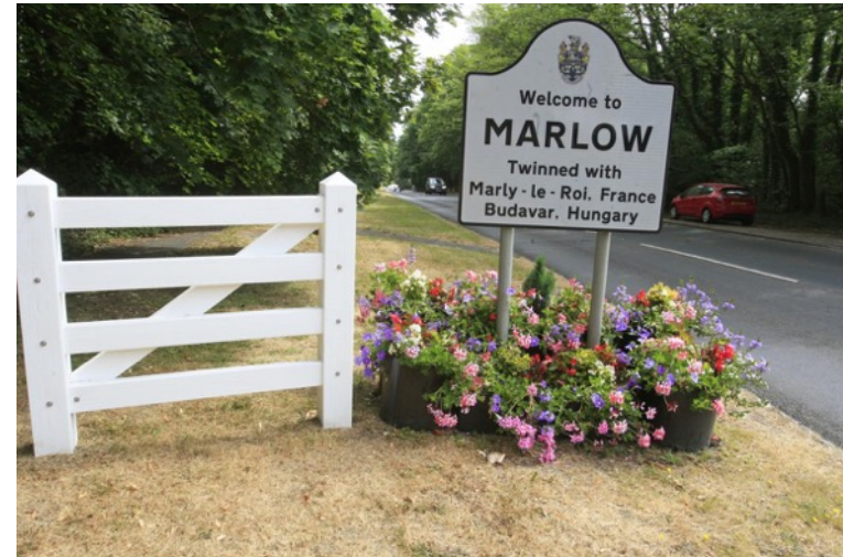
Figure 11: Village entrance with planting, signage and fencing installed in Marlow to deter speeding. Marlow, Buckinghamshire. Source: www.bucksfreepress.co.uk .
