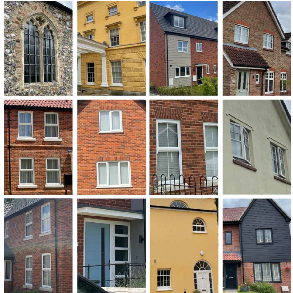
Figure 32: A variety of Rackheath quality windows, gives character and interest to the streetscape. Common types include mock sash windows, single and double hung windows, casement windows, shaped windows. Source: own.
