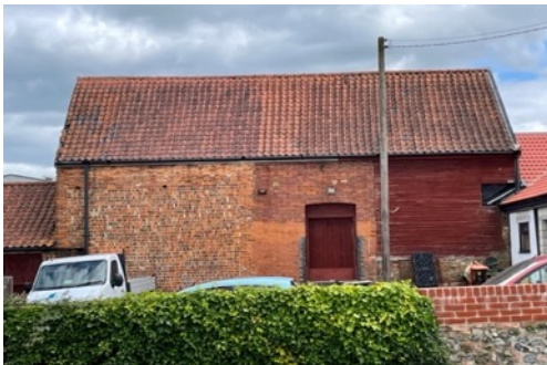
Figure 16: Red brick barn on Green Lane West, showing old red brick. Rackheath. Source: own.
